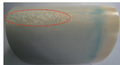
图10 零件底部贫胶区 Fig.10 Schematic diagram of poor glue zone at the bottom of the part
